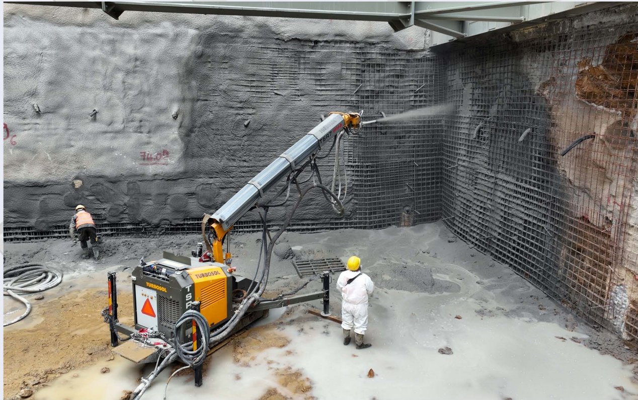
Shotcreting at the 8th level of AKADIMIA Station.
