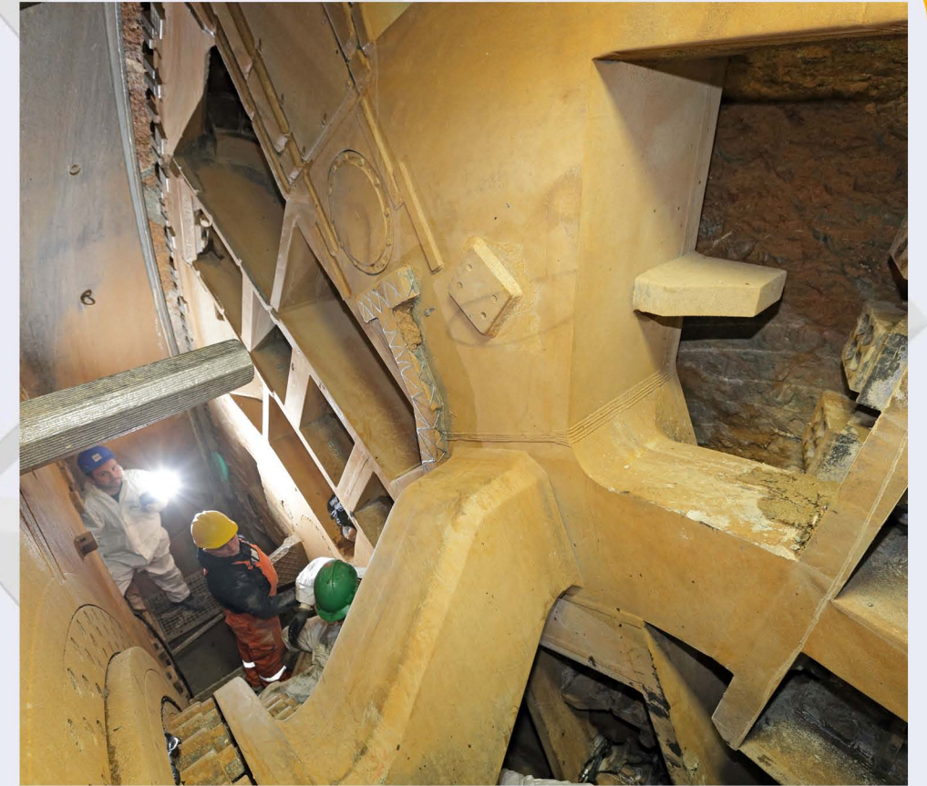
Maintenance works inside TBM "ATHENA" excavation chamber.
