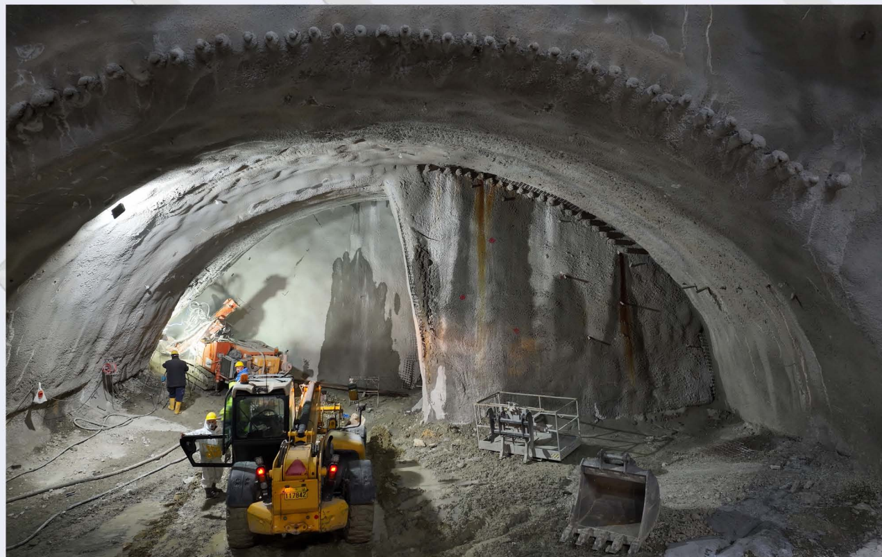
Excavation of NATM tunnel - DIKASTIRIA Station.
