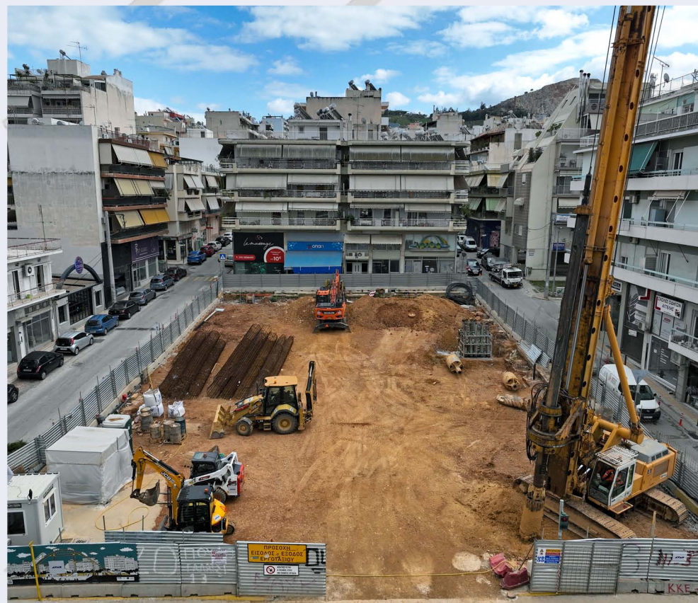
Construction of piles at the central trench of ALSOS VEIKOU Station.
