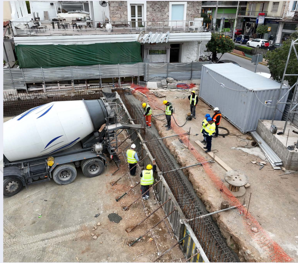
Concreting of the pile cap beam – KESSARIANI Station.
