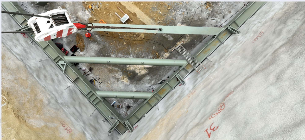
Works for the installation of struts at AKADIMIA Station.
