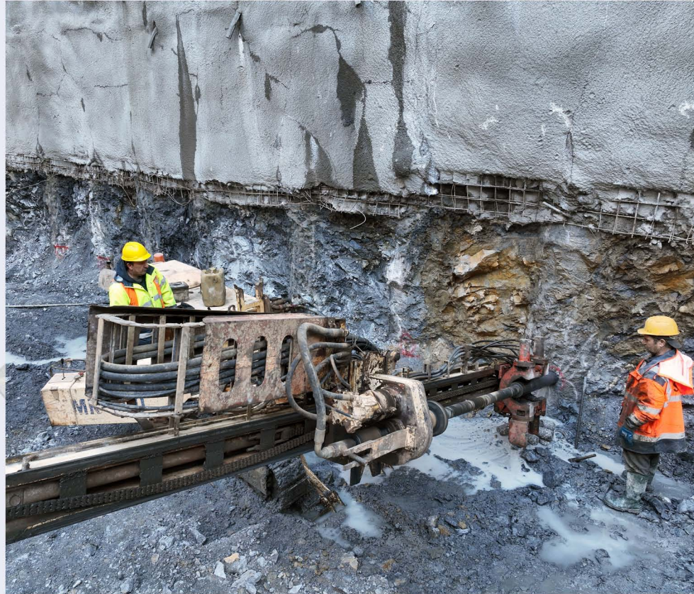
Drilling of anchors – KOLONAKI Station.
