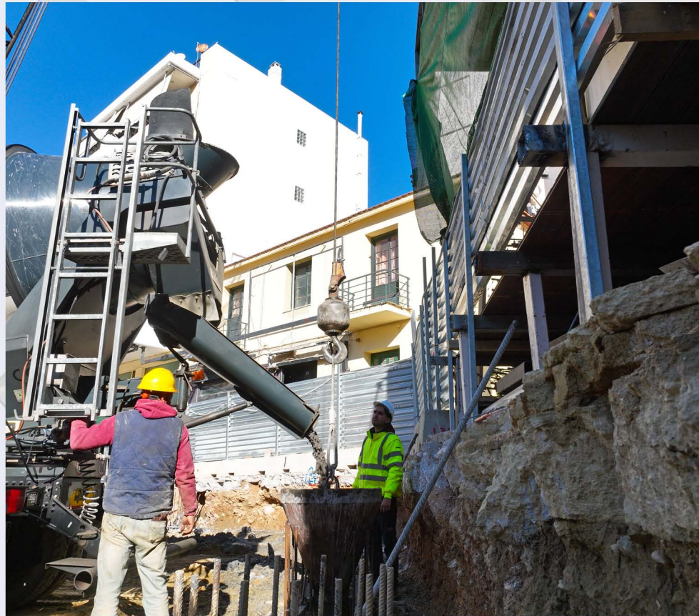
Concreting of piles – KESSARIANI Station.
