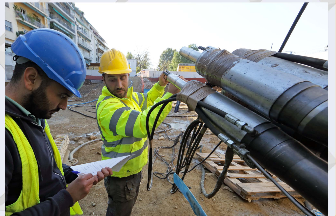
Anchor tensioning process – EVANGELISMOS TRUMPET Shaft.
