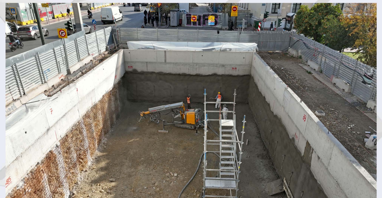
Excavation at Vivliothiki Shaft.
