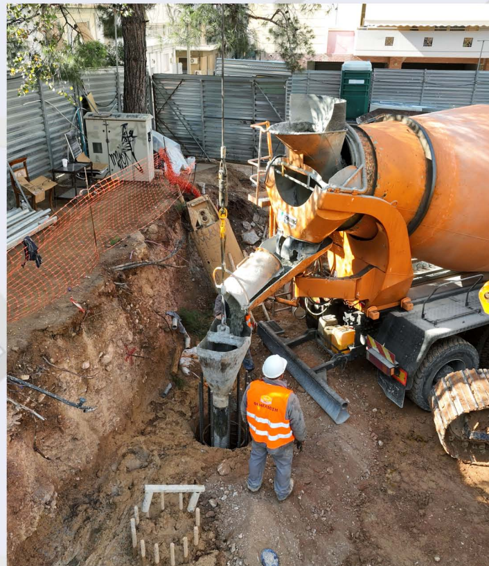
Concreting of piles – ILISSIA Station.
