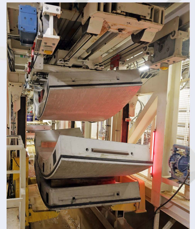
Transportation of precast rings inside the TBM.
