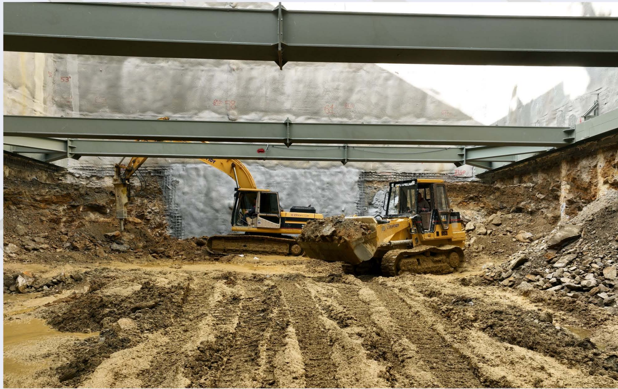
Excavation of the 7th level – AKADIMIA Station.
