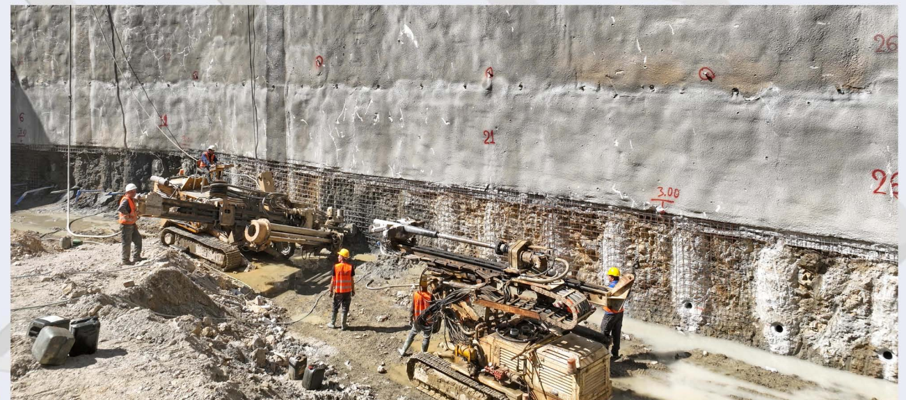
Excavation of the 3rd level at KOLONAKI Station.
