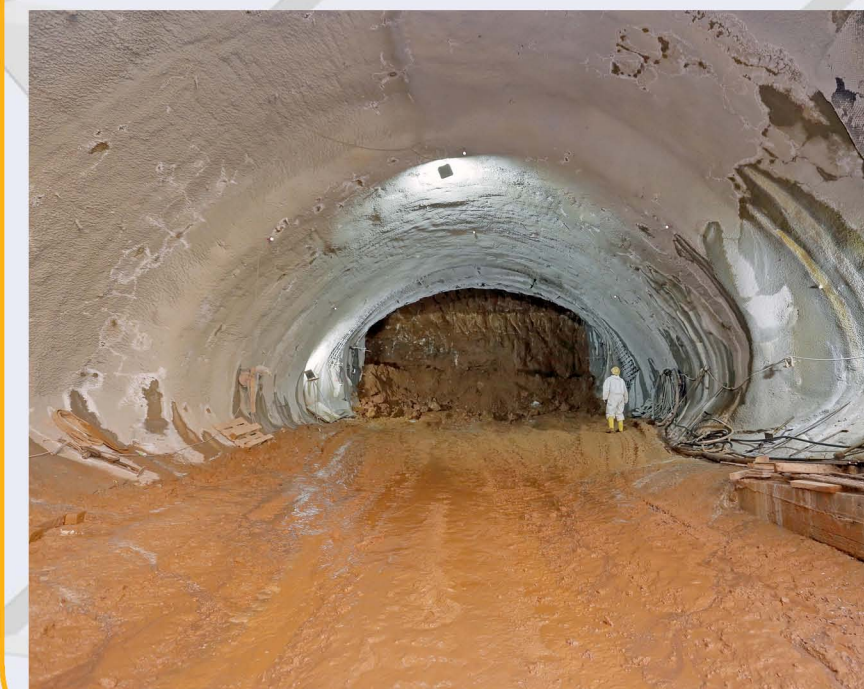
Excavation of connecting gallery – GNA shaft.
