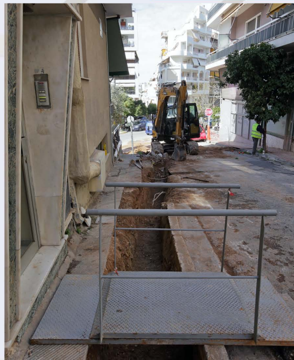
Network diversion works at ILISSIA Station.
