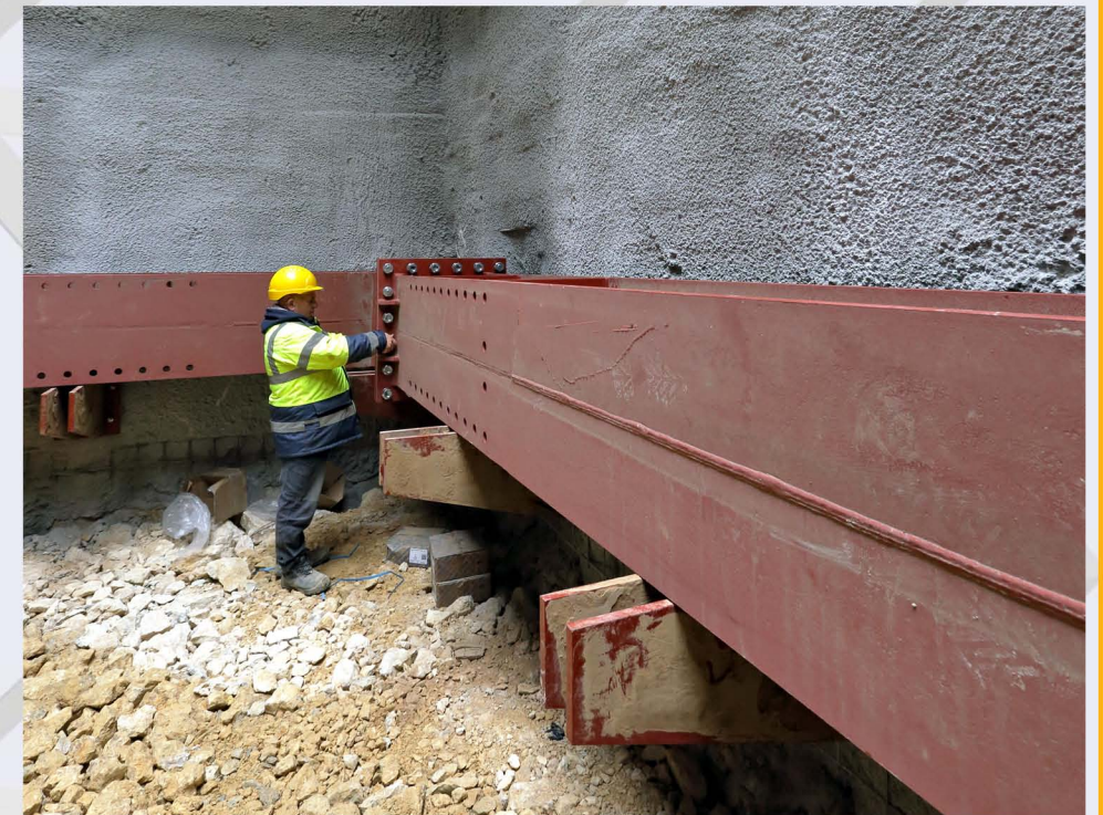
Installation of 3rd level struts at EYDAP shaft.
