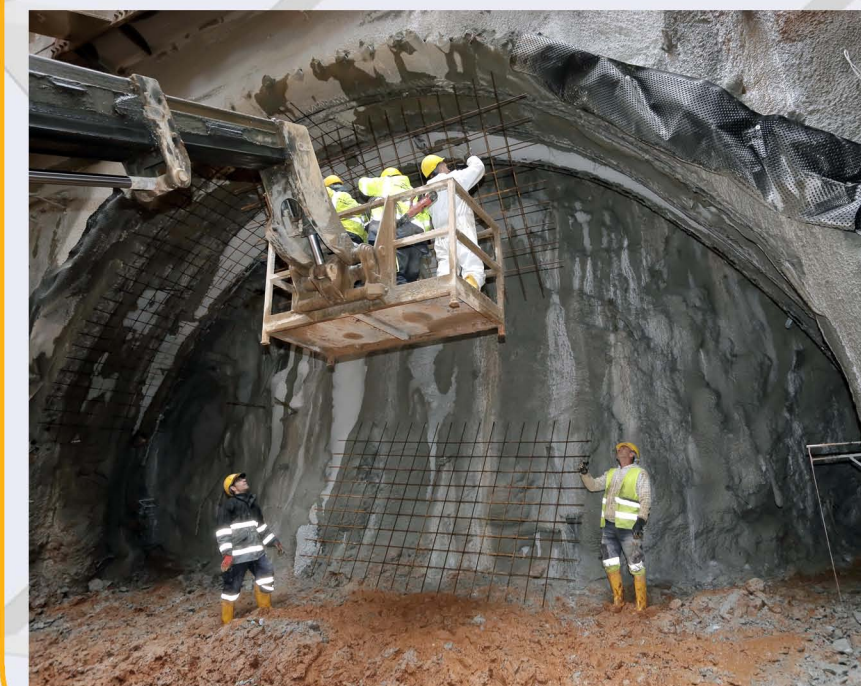
Installation of frame at the connecting gallery – GNA shaft.
