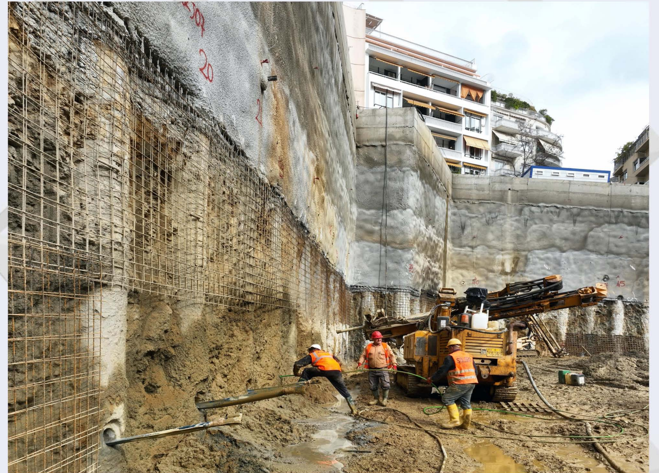
Drilling of 3rd level anchors in KOLONAKI Station.
