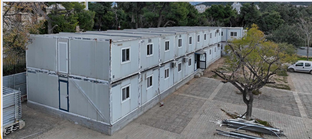
Worksite installation works in DIKASTIRIA Station.
