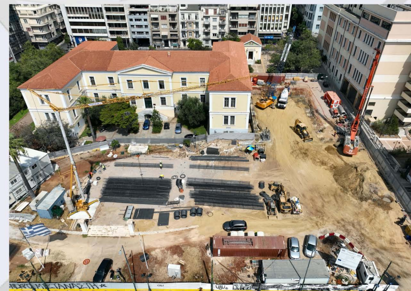
Drilling and construction of piles at AKADIMIA Station.
