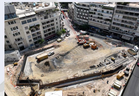
Drilling and construction of piles at KOLONAKI Station.
