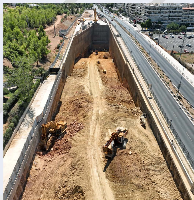
Excavation at Veikou TBM Shaft.
