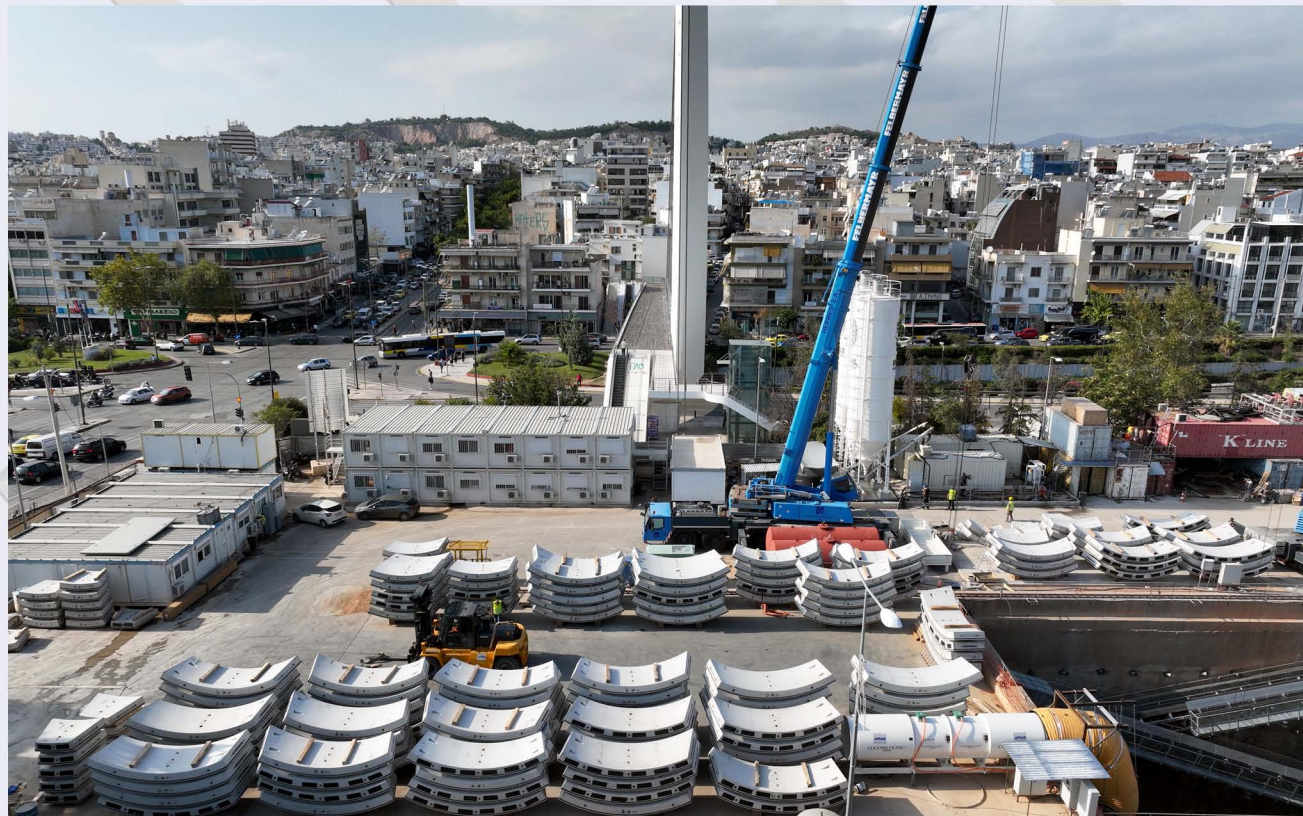
Arrival of tunnel segments in Kاتهaki TBM Shaft.
