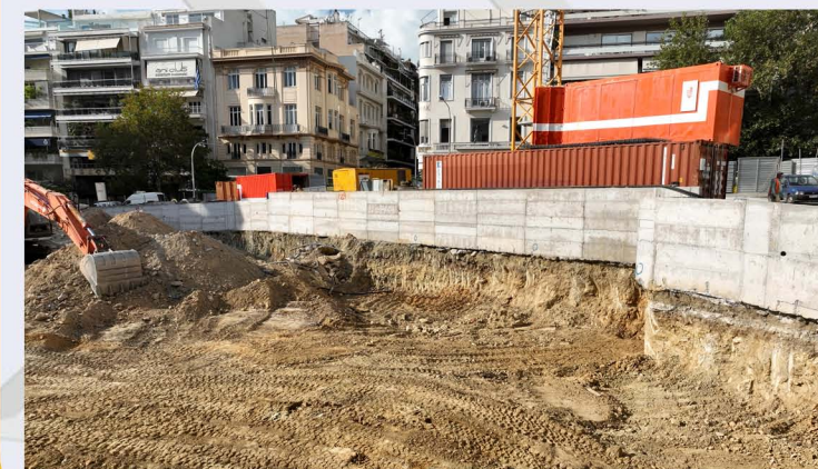
Excavation of the 1st level in KOLONAKI Station.
