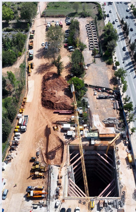
Completion of excavation works in GNA Shaft.
