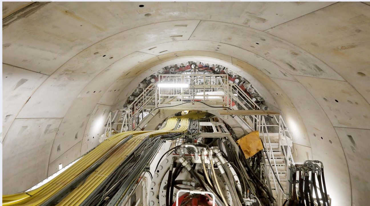
Lined tunnel through "Athena" TBM machine.
