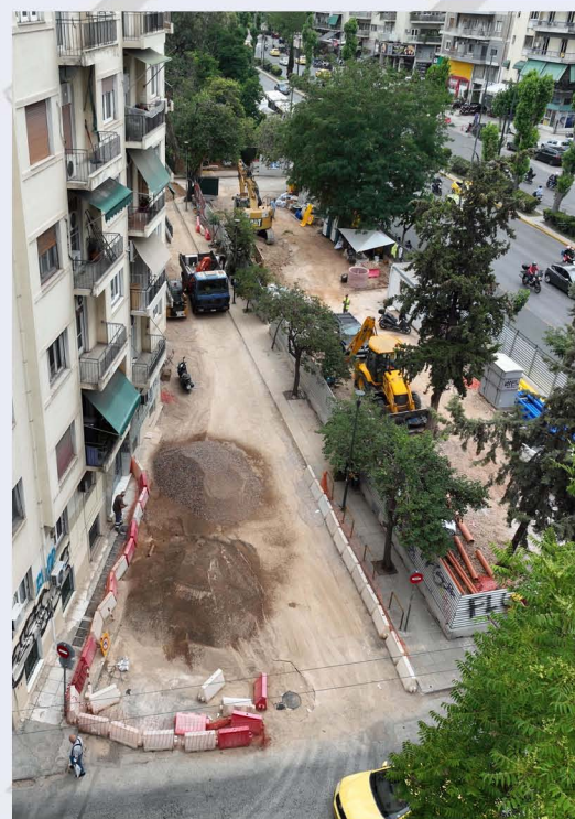
Network relocation works in ALEXANDRAS Station.
