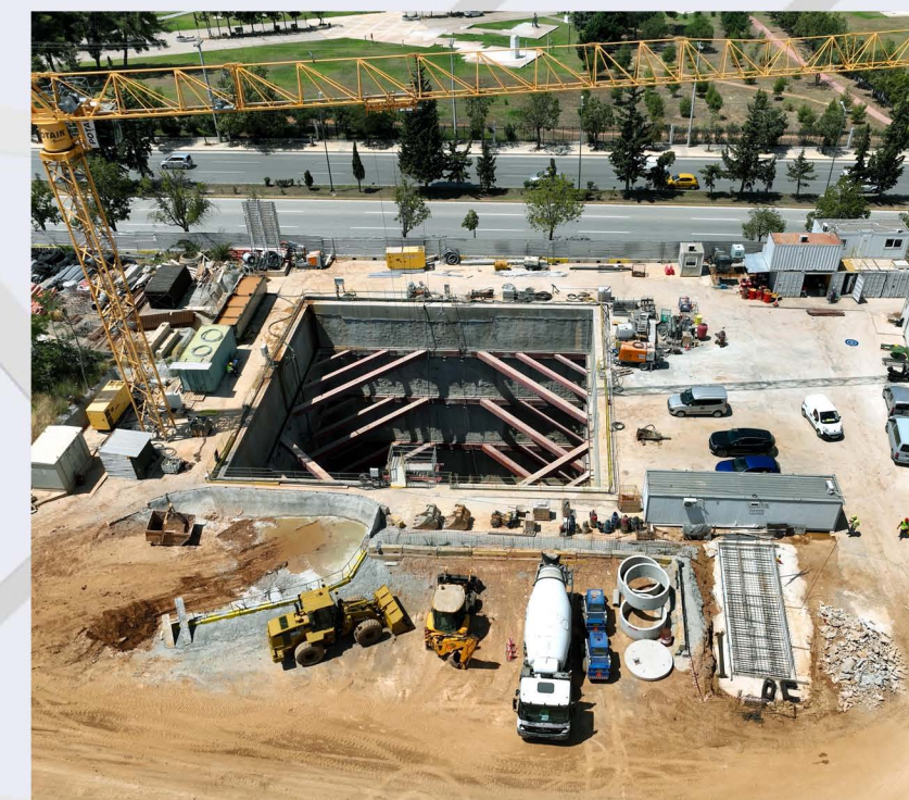
Excavation in progress at GNA Shaft.
