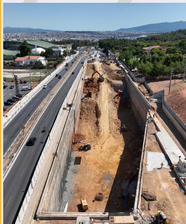
Excavation in progress at Veikou TBM Shaft.
