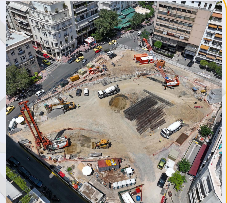
Drilling of poles – KOLONAKI Station.
