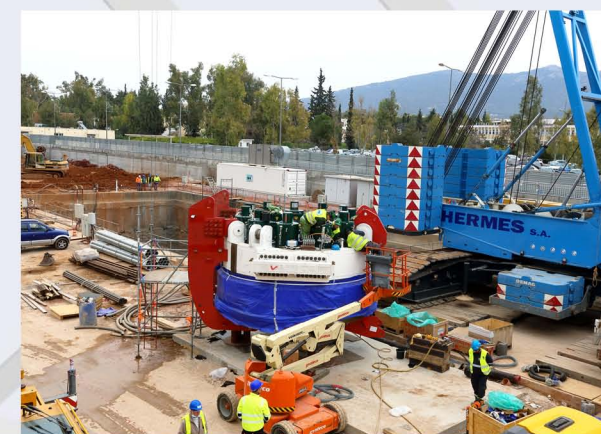
TBM assembly.
