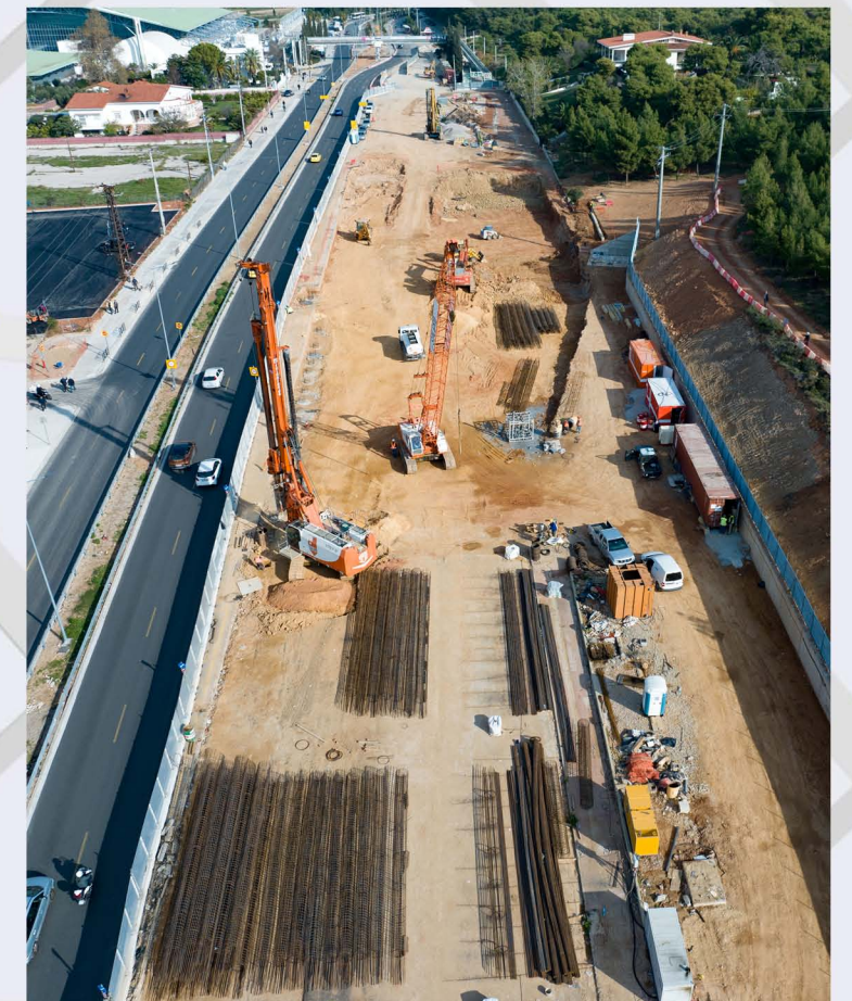
Pile drilling in TBM Veikou Shaft.
