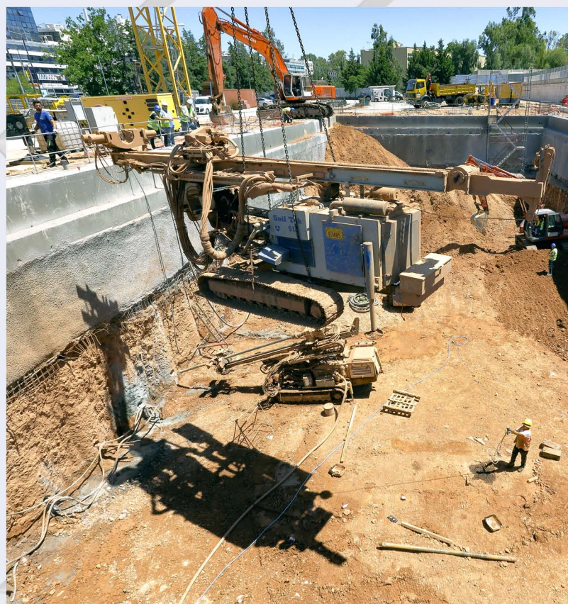
Arrival of perforating equipment for the construction of anchors in KATEHAKI TBM Shaft.
