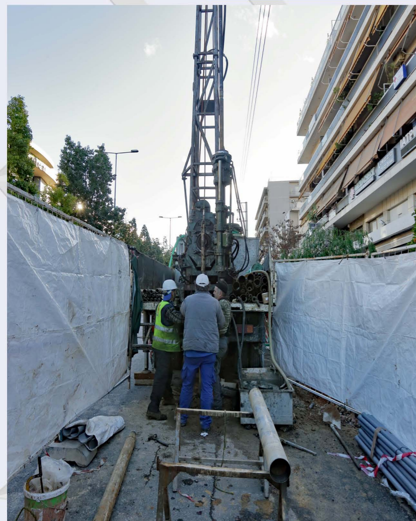
Borehole in progress.
