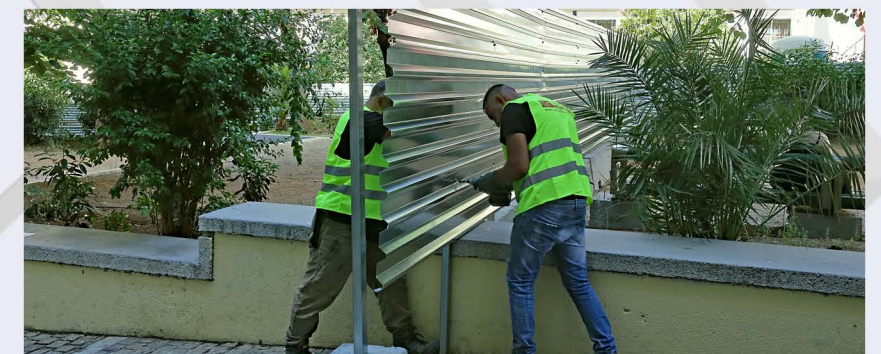
Installation of metal sheets at Evangelismos.
