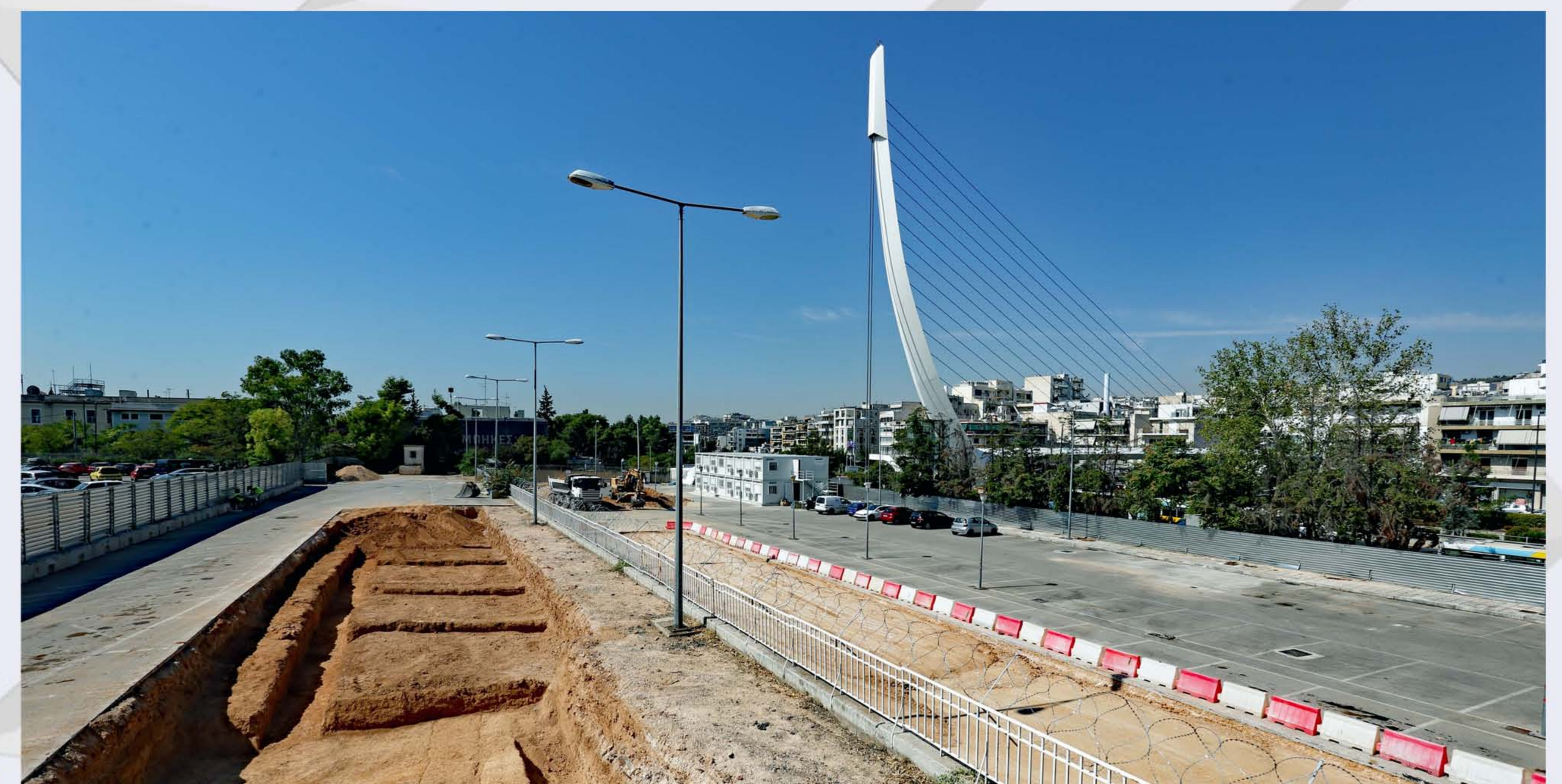
The first worksite of Line 4 A .
