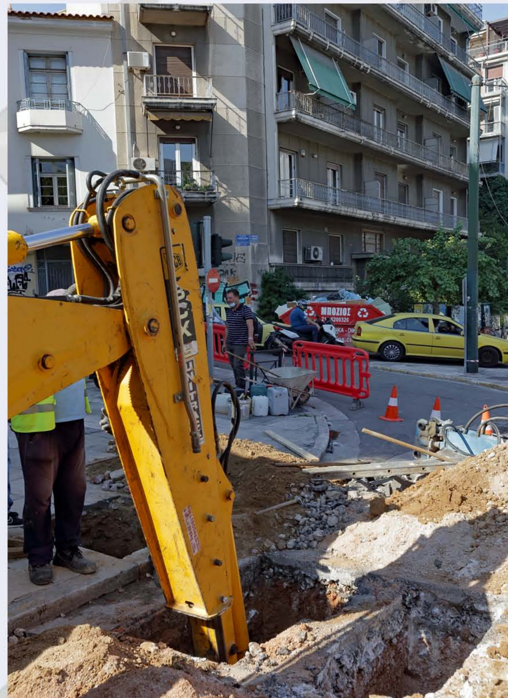
Works for the relocation of PUO networks in Alexandras Avenue.
