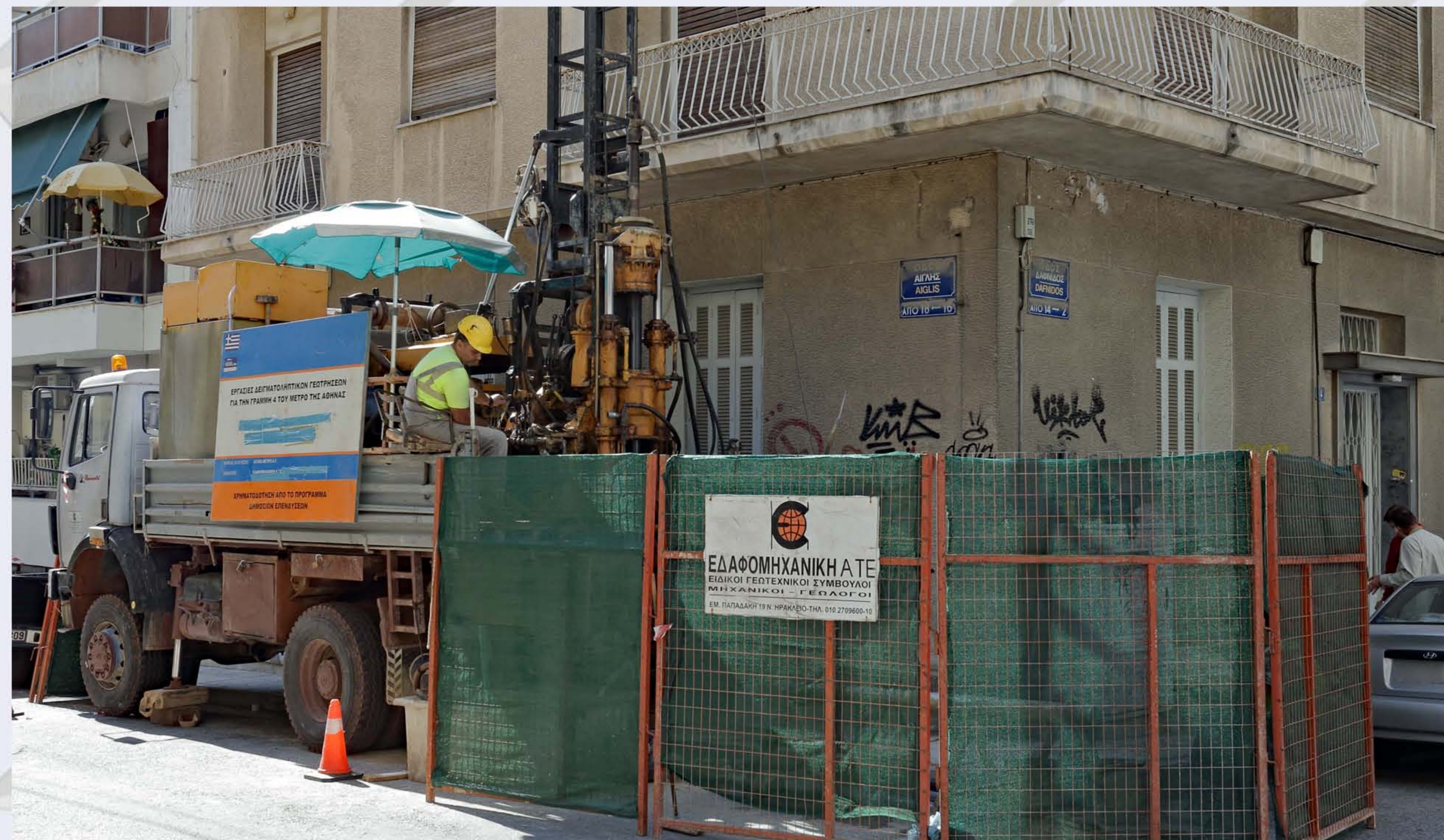
Borehole in progress.
