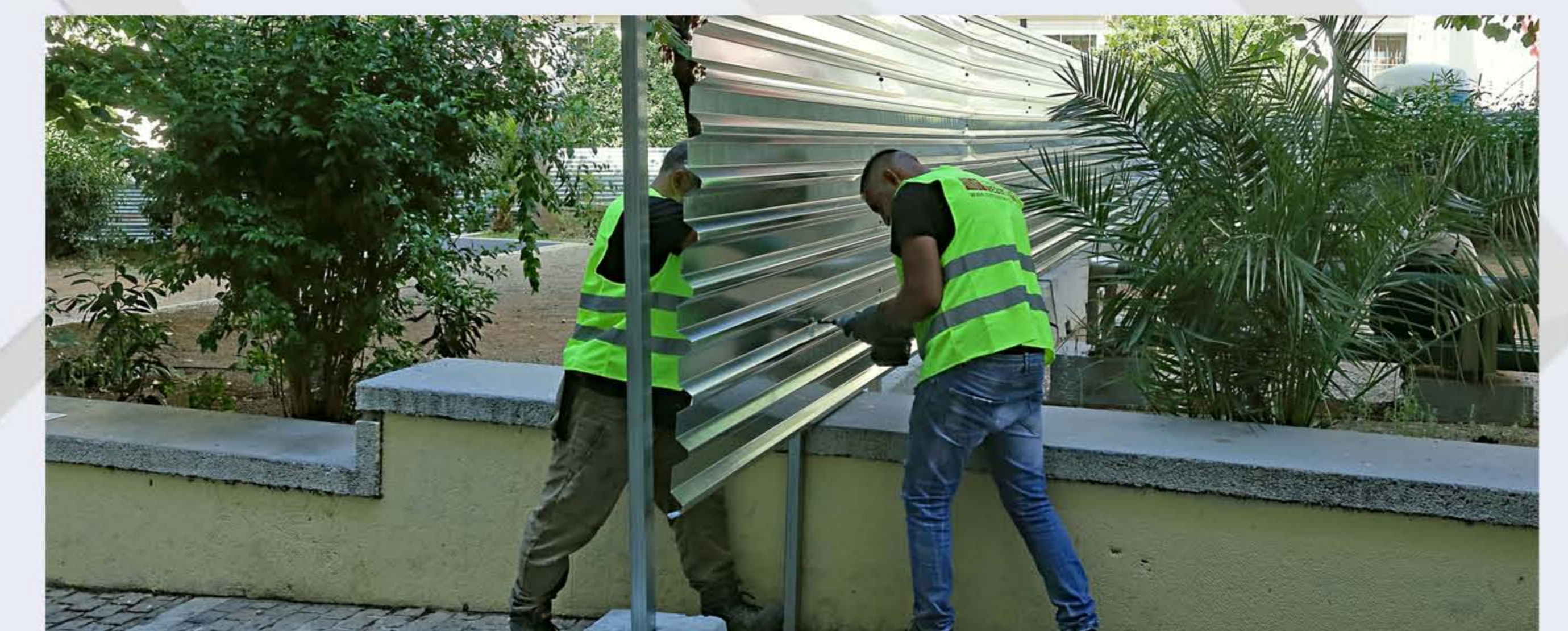
Installation of metal sheets in Evangelismos.
