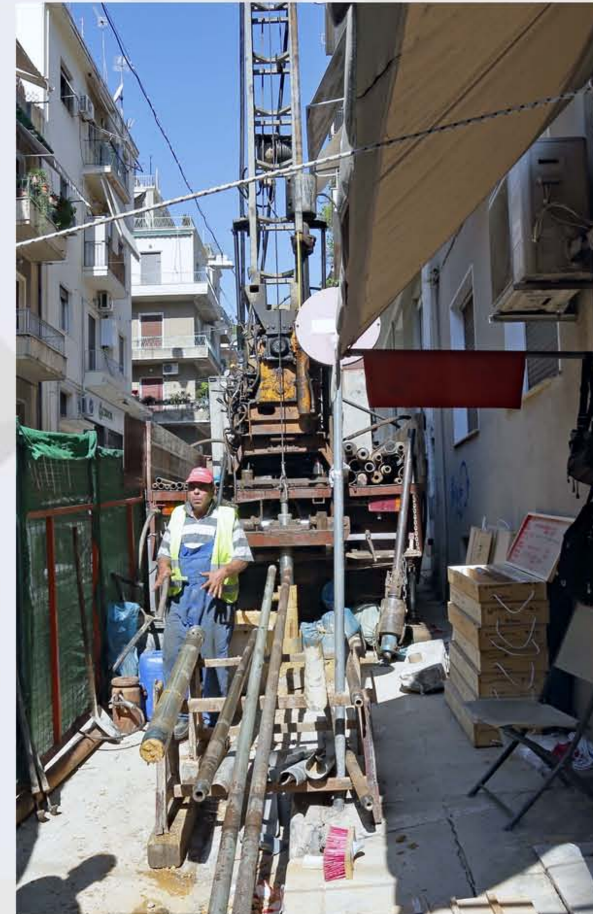
Sampling drilling rig.
